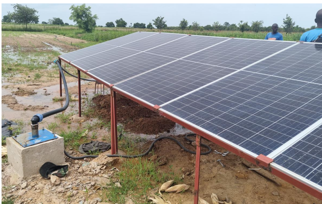
Participants of the curricula development at the demonstration site of CSA and CIS at Daga Birame et Kafrine in Sénégal where groundnut, cowpea and millet are under evaluation and also the use of pv for water pumping for irrigation will be using in the near future.
